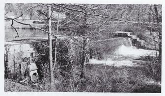
aesthetic and recreational purposes. Although a penstock was installed for possible hydroelectric generation, it has never been equipped with a turbine or generator.
