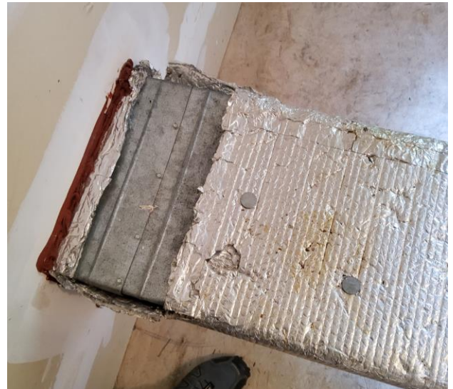
Inadequate insulation on ductwork
