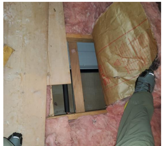
Attic floor with no air barrier between acoustic ceiling and attic space
