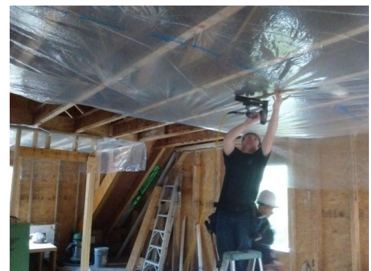
Smart vapor retarder membrane stapled to attic floor joists (photo credit: Fine Homebuilding)
